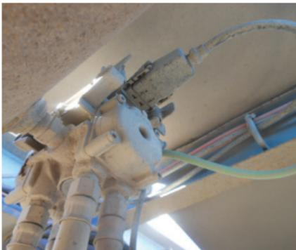
Do not overtighten wires onto air hoses with tie wraps; this may cause wire pinching as hoses expand.
